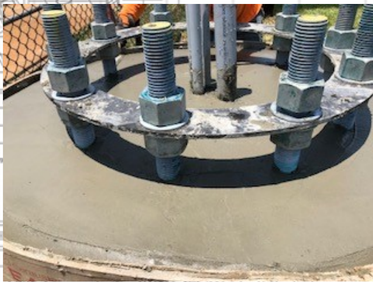
Mercer Stadium – Light Masts Replacement
