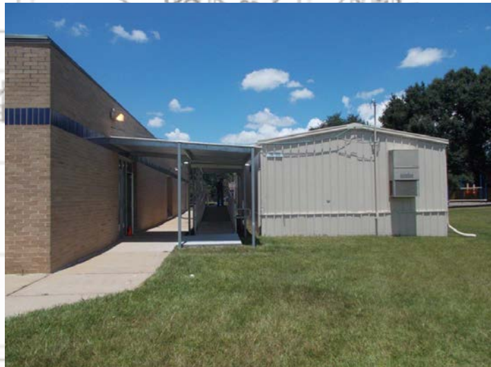
Temporary Building Relocation - 2018
